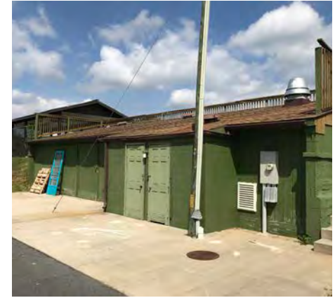
Pump house and maintenance area
