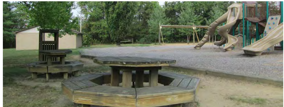
View of permanent restrooms in Town Park, with 'back' turned to playground - entrance is on opposite side from playground
