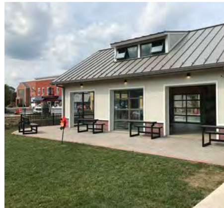
Market Pavilion paver patio
