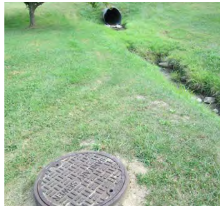
Sanitary sewer near drainage swale
