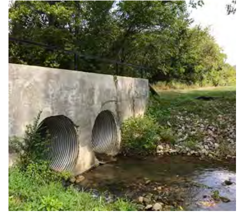
Bridge culvert over Town Run
