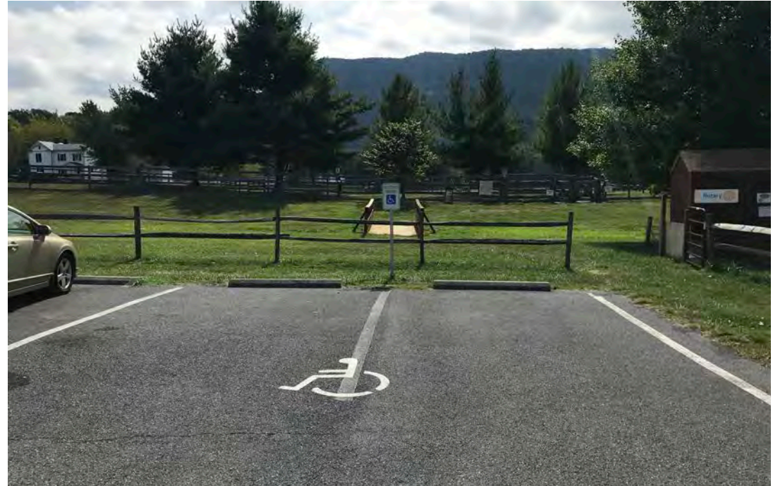
ADA Accessible parking at Town Park in one of the asphalt paved parking lots, an accessible route is needed to tie parking spaces to park features
