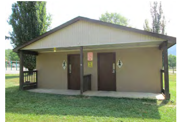
No accessible route to restroom facilities
