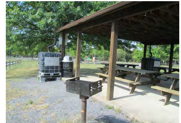
Moose Lodge Park Shelter with rainwater harvesting
