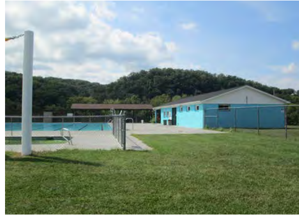
View west toward the pool house
