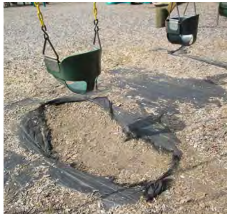
Safety surfacing not in compliance
