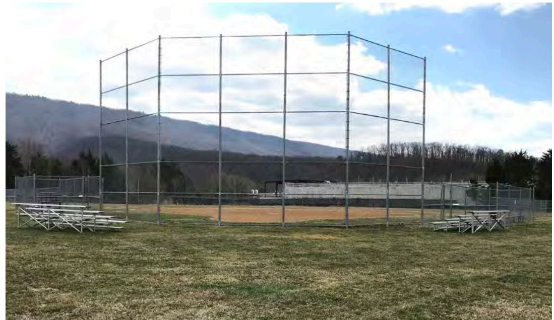
Existing diamond fields at Town Park
