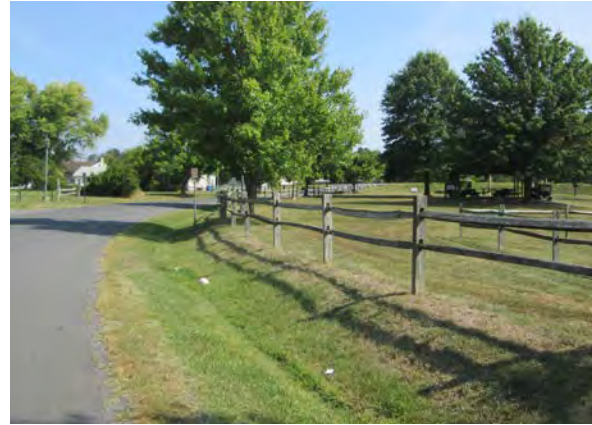
Drainage swale along Park Road
