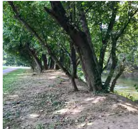
Eroded river bank lacking ground cover
