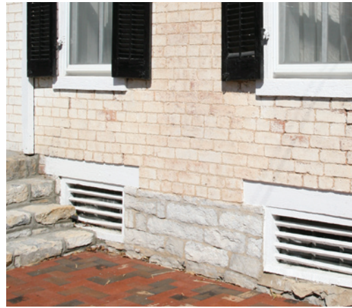
Stone provides the foundation for many of Strasburg's earliest buildings.
