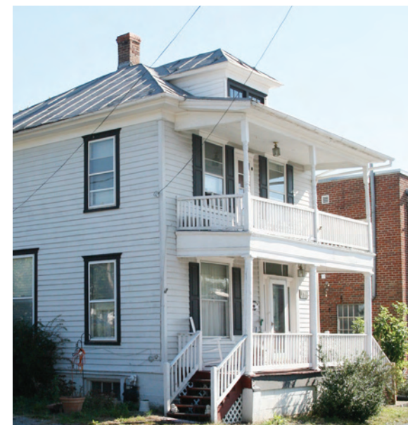
A two-story porch on this two-bay American Foursquare gives it a more vertical appearance than typical examples of this style.
