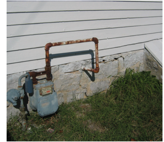
Evergreen plantings could help screen the gas meter from view while allowing access for the meter reader.
