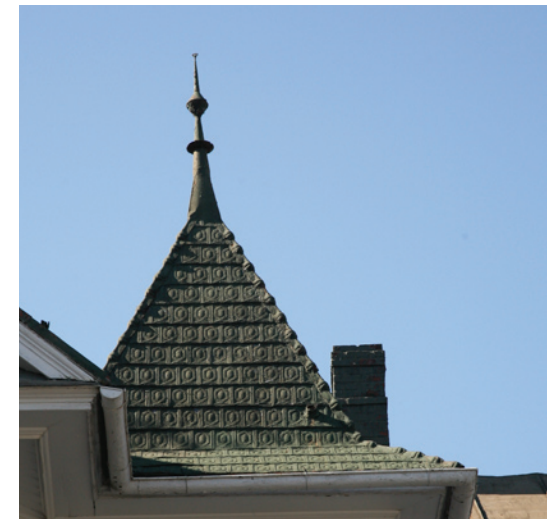
This metal-shingle-clad tower roof terminates in a round ball finial.
