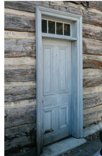
Another early door opening with a four-light transom and a four-panel door.
