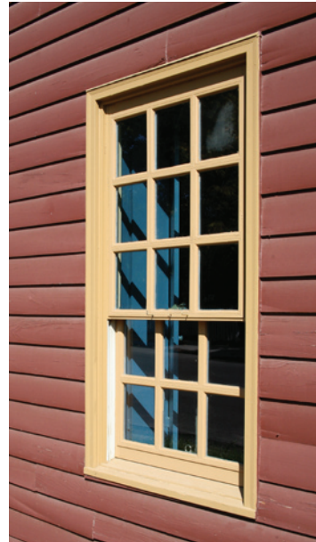
Early windows had many small panes of glass as seen in this nine-over-six example.
