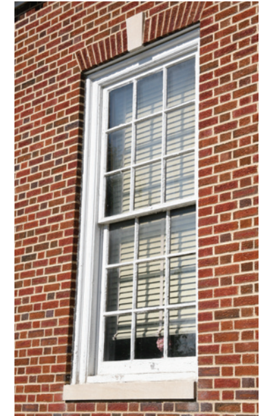
The Colonial Revival style made small-paned windows popular again in the early twentieth century.
