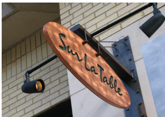
In some cases, it may be possible to attach a lighting source to the sign bracket.
