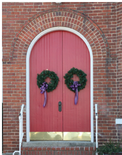
The arched doors are composed of vertical boards and fit the arched opening.
