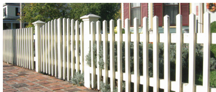
This fence, with its widely spaced pickets, suggests a sense of enclosure but is visually open.
