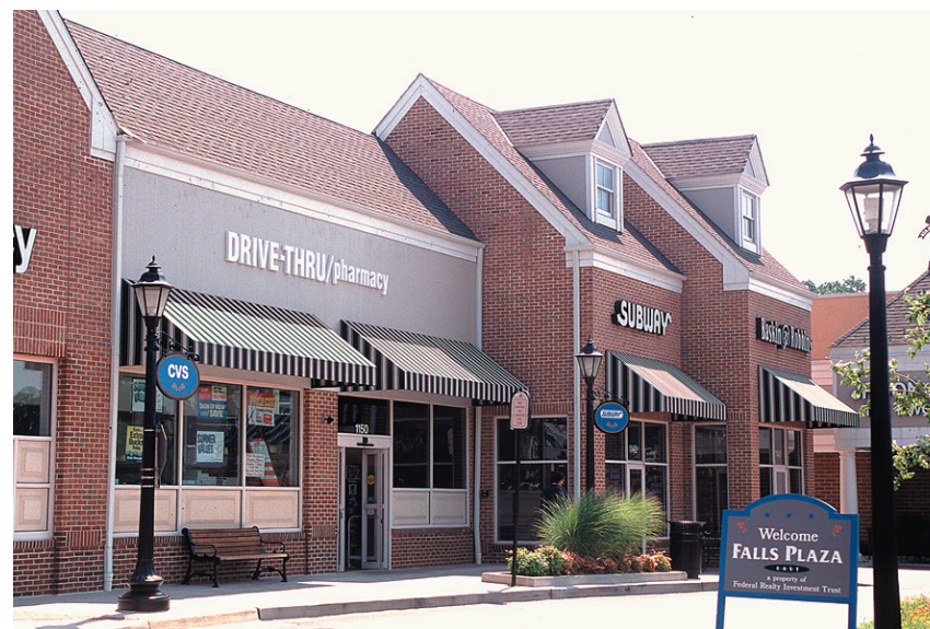
This more contemporary development is based on traditional commercial building elements and uses many of the principles covered in the New Construction chapter. With its storefront windows and awnings, this type of design may be appropriate for parcels zoned highway commercial such as those in the Hupp's Hill district.
