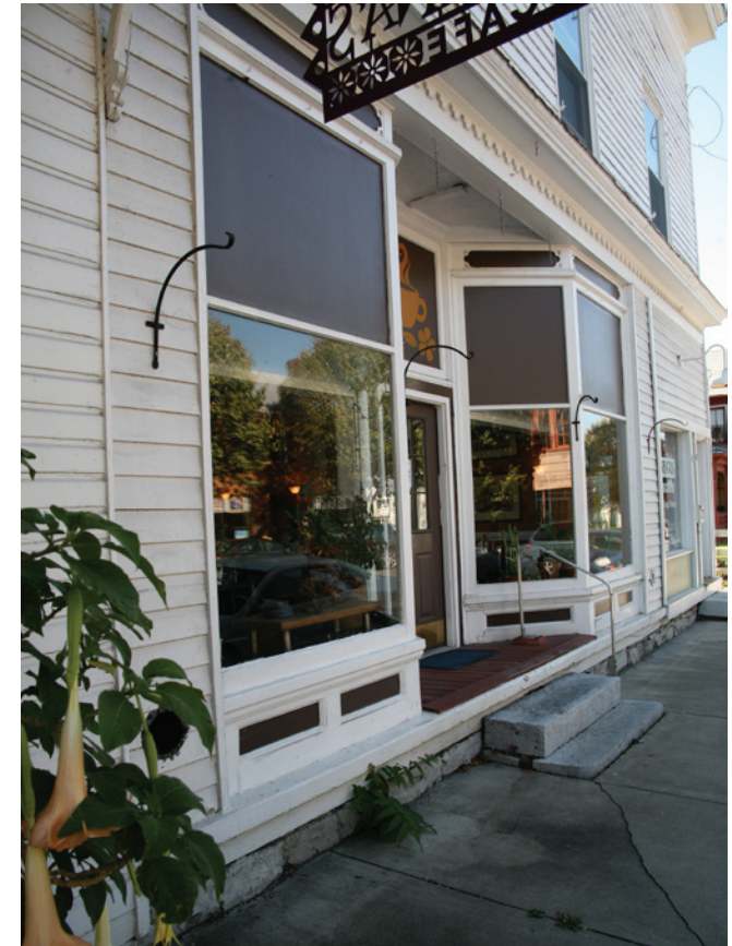
Recessed entries and large plate glass windows resting on wooden bulkheads, and capped by decorative storefront cornices are typical of Strasburg's historic commercial structures from the late nineteenth and early twentieth centuries.
