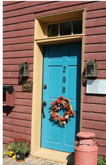
An early doorway with a three-light transom and six-panel door.
