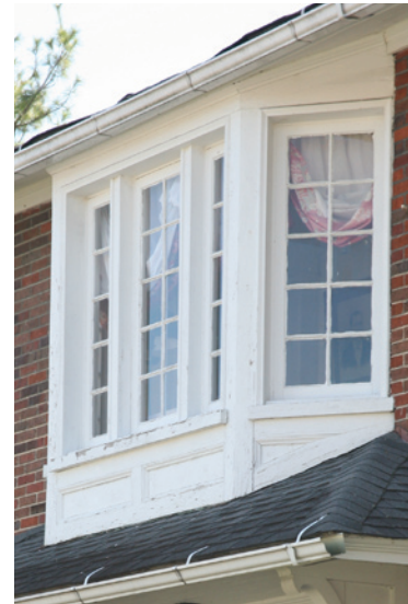
Small-panes were also used in casement windows as seen in this bay window example.
