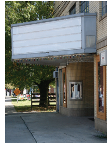
The metal marquee of the Strasburg Theater appears to be an original feature of the building.
