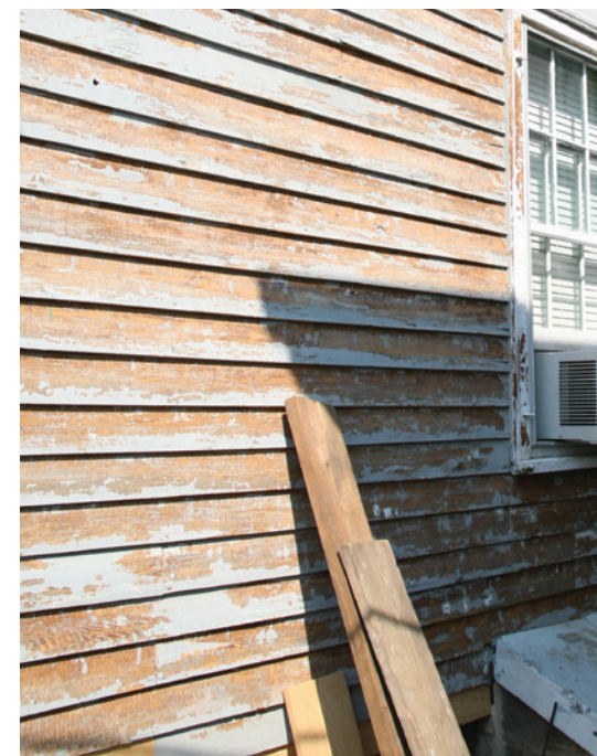
Fully scraped, this surface is ready for final sanding, the appropriate primer, and paint.
