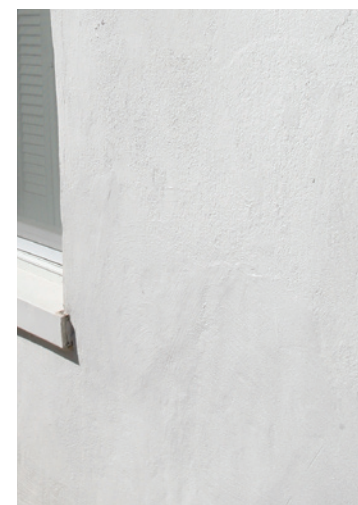
Smooth-finished stucco may provide a more elegant appearance and was often scored, historically, to resemble stone.
