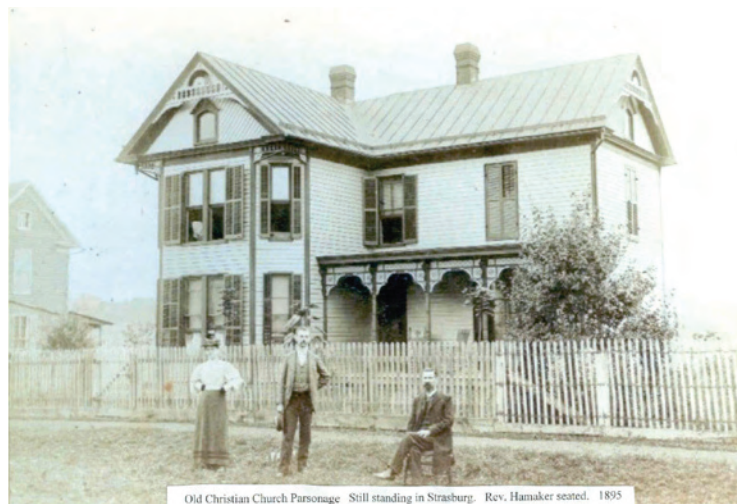
Historic photographs, such as this 1895 view of the Christian Church parsonage, often can aid homeowners in restoration efforts. Victorian era residences often lose their detailed woodwork over time due to deferred maintenance. These images can also be a guide for the application of paint colors, roof materials, and site features.
