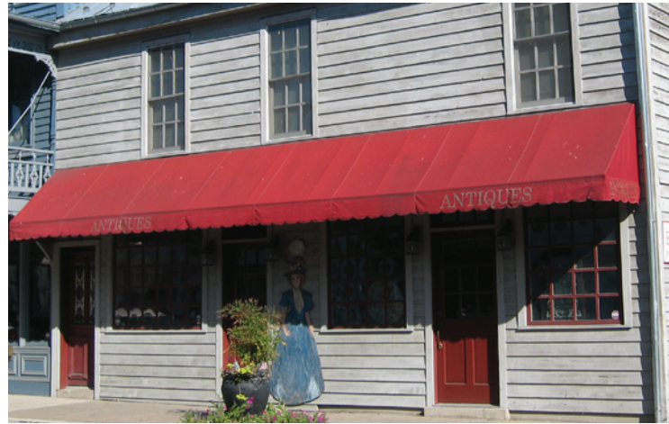
This sloped fabric awning is fixed in place and has discreet lettering on the scalloped valance.
