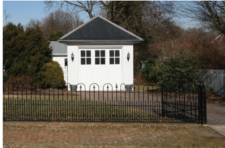
This one-car garage is located at the rear of the lot facing the street. The garage door has a popular early-twentieth-century design that appears as three doors each with four lights above two vertical panels
