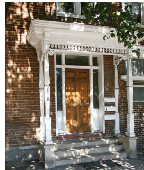
This Victorian-period entry porch is notable for its beautifully detailed woodwork.
