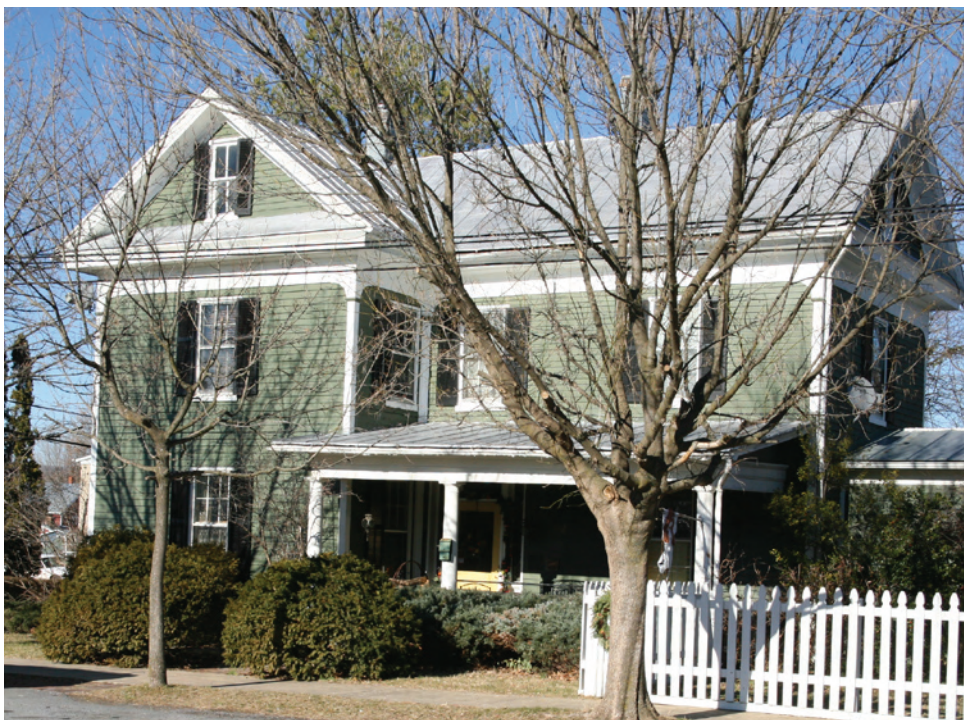
This L-gable vernacular Victorian has many elements typical of the style. A deep cornice or frieze below the eaves and decorative brackets where the cornerboards meet the cornice are local vernacular elements.
