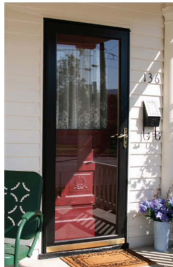
A full-reveal storm door allows view of the original Victorian period partially glazed door.
