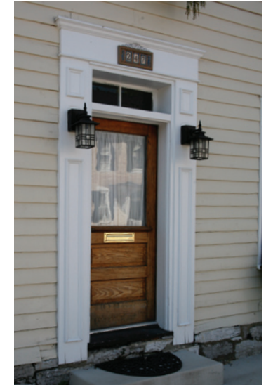
A classically ornamented door surround with a two-light transom and a partially glazed door.
