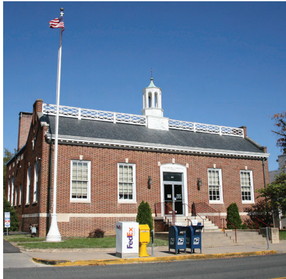
The U. S. Post Office, built ca. 1936 at 152 W. King Street, is Strasburg's best example of this style. Decorative elements include cast stone keystones over the nine-over-nine double-hung sash windows, a rooftop balustrade and cupola, and a delineated water table.
