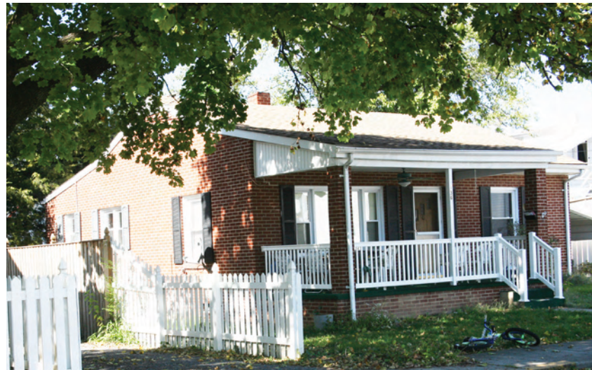
A small Ranch-style, this variation has a partial width porch with brick columns. The porch roof is a continuation of the main roof line, a feature seen in the earlier Bungalow style.
