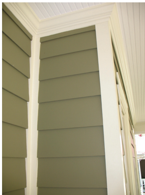
Inside and outside cornerboards, crown molding, and beaded-boards suitable for a porch ceiling are some of the trim details available in substitute materials for new construction.
