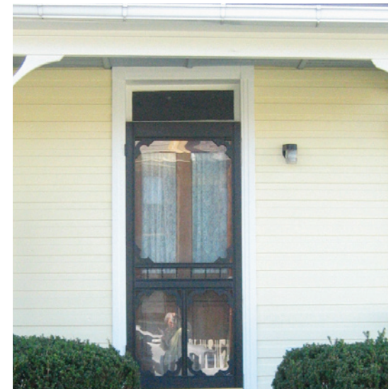
Storm panels replace the screen in this example of a Victorian-embellished screen door.
