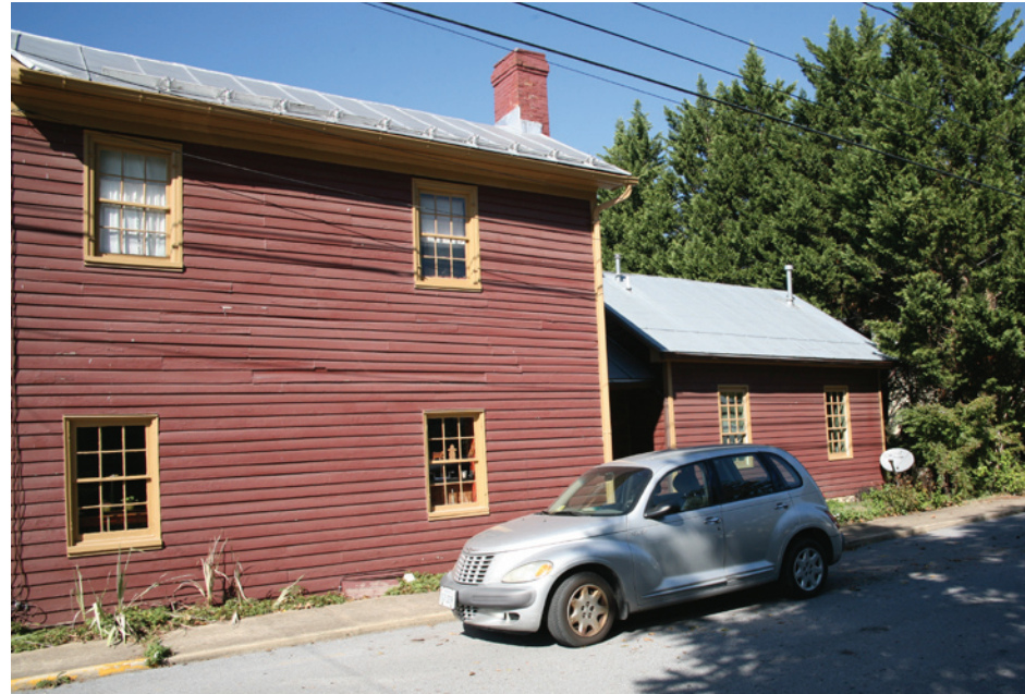
The one-story addition is attached to the main structure by a hyphen. The smaller scale of the addition does not detract from the main structure.
