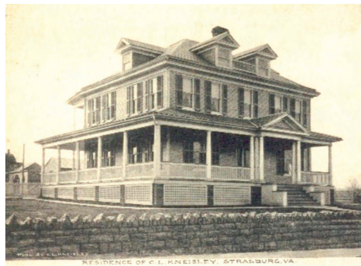
This view of the C. L. Kneisley House, built by the owner of the local drug store in the early twentieth century, shows a rough-faced, coursed stone wall with jagged top course, a common Strasburg feature.
