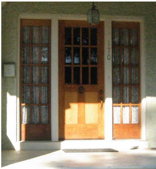
Note the multi-pane sidelights that echo the pane division of this door.
