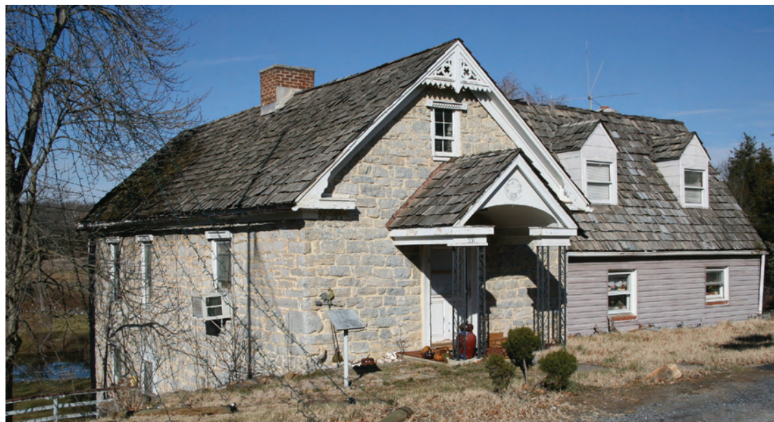
This stone bank house is known as Frontier Fort or Hupp House. Constructed in the mid-eighteenth century, the frame wing, entry porch, and decorative woodwork are later additions.
