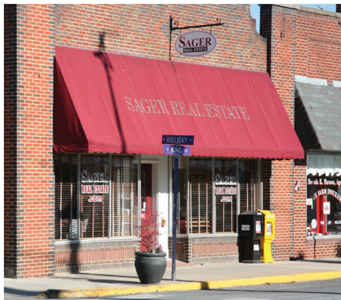
Fabric awnings are appropriate for downtown buildings.
