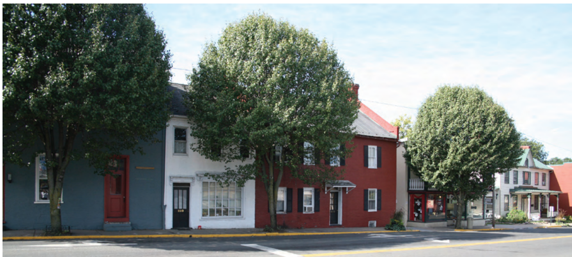
At the eastern edge of the district, this row of structures on East King Street, just west of its intersection with Massanutten Street, represents the mid-nineteenth-century commercial development of King Street after the realignment of the Shenandoah Valley Turnpike in 1842.
