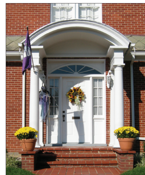
Classical details were used for the design of a portico that echoes the fanlight over the front door.
