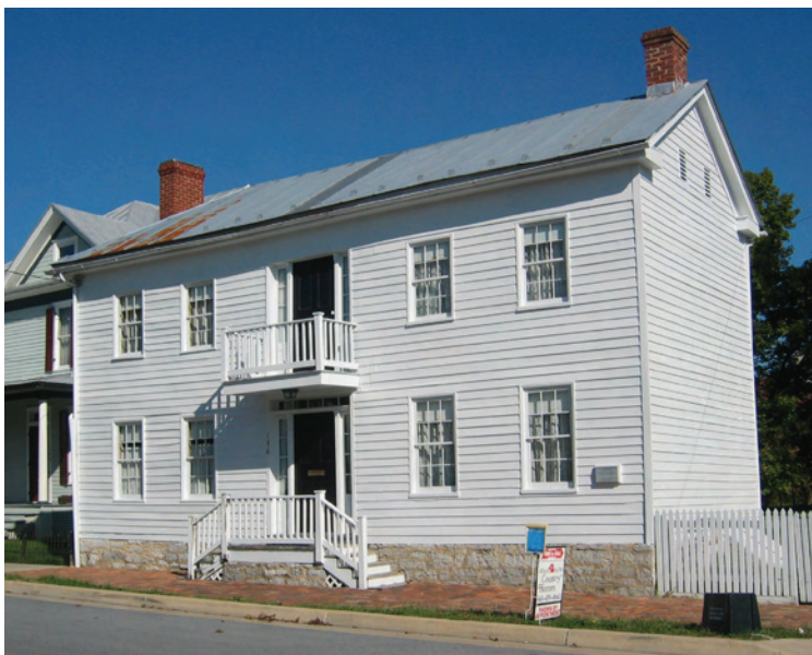
This five-bay frame Federal residence sits on a native limestone foundation and has chimneys at each end of the structure. A rectangular transom and small-paned sidelights frame the door. The one-bay upper story gallery shelters the entrance. Note: During rehabilitation it was discovered that the first floor on the left side is the original log dwelling from which the house later expanded.
