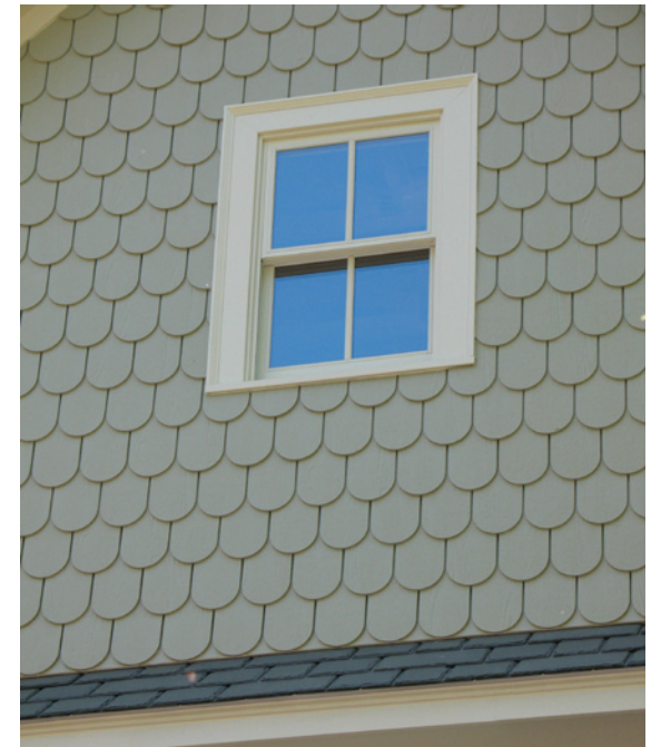
Historic shingle patterns are available in cementitious siding products.
