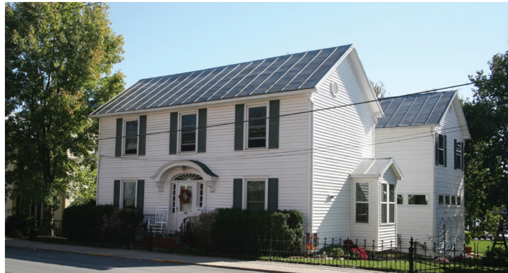
The two-story addition to the rear of the historic residence echoes its scale but is differentiated from the older structure by the size and placement of windows on the first floor level.
