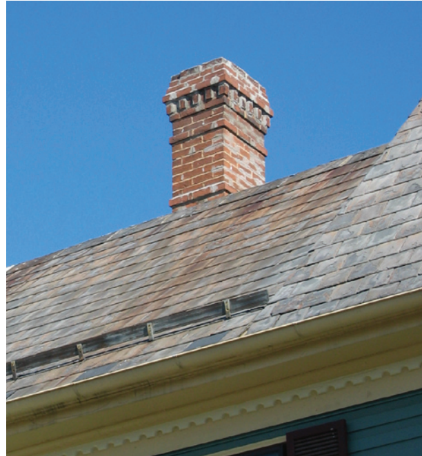
Late-nineteenth residences often incorporated centrally located chimneys with details such as the belt courses and corbeling seen here.
