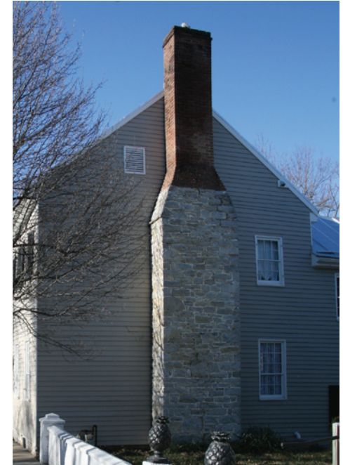
Exterior-end chimney constructed of a stone bottom portion and brick upper portion are found throughout the Shenandoah Valley.
