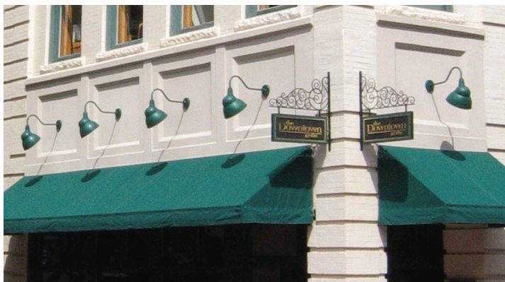
Gooseneck fixtures provide a shielded light source for the awning and signs for this restaurant.
