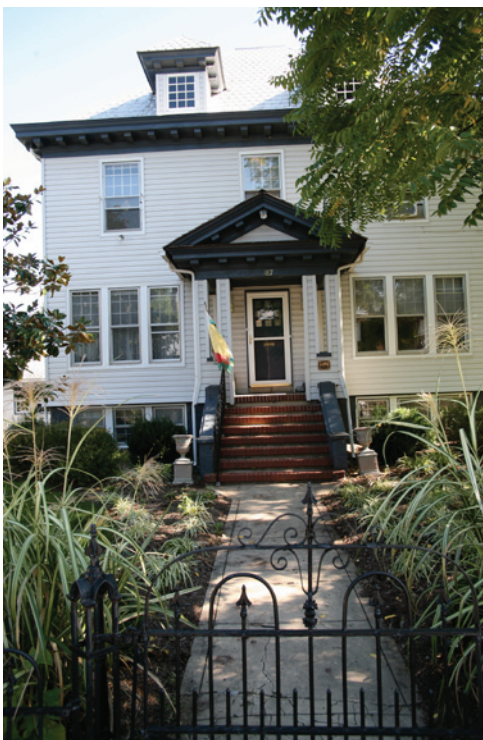
Scored concrete is also a popular walkway material and is often associated with walkways installed in the early twentieth century or after.
