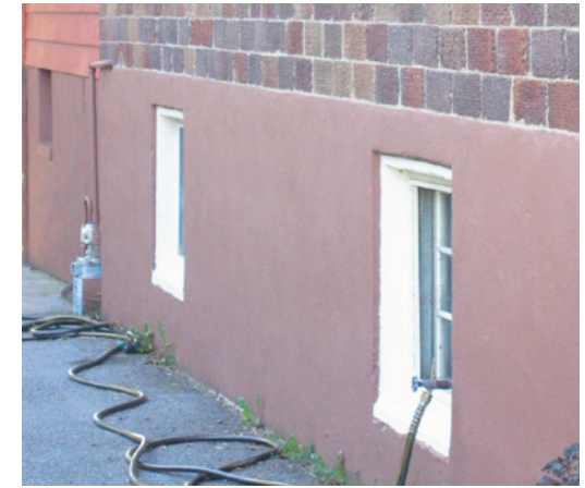
Stuccoed or parged foundations are also found in the district.
