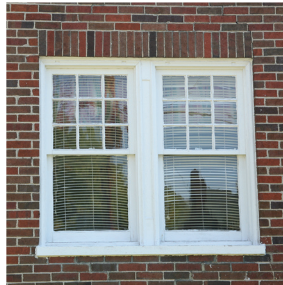
Popular window designs in the early twentieth century often featured multiple panes in the upper sash and a single pane in the lower sash.
