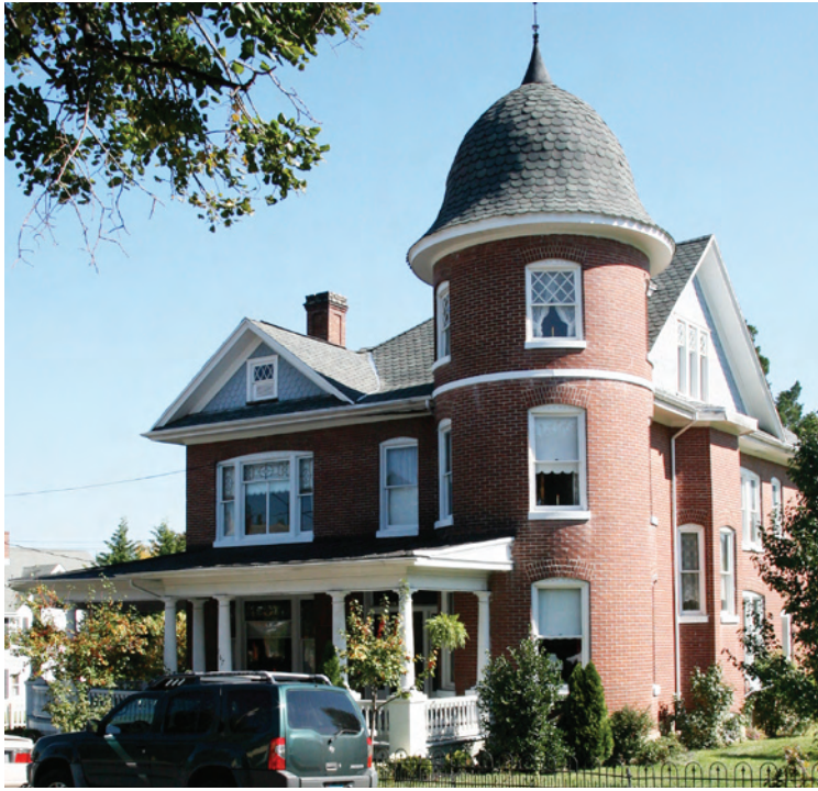
This local example of the Queen Anne style has decorative shingles and diamond-paned divisions in the upper sash of the third floor windows. The turret on the dominant tower is capped by an S-shaped roof and finial.
