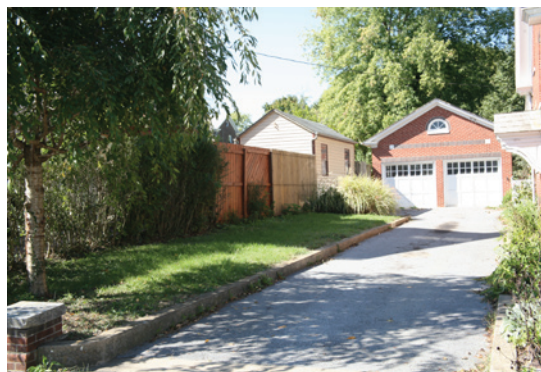
An asphalt driveway, with brick piers at the sidewalk and concrete curbing along its length, leads to a historic double garage.
