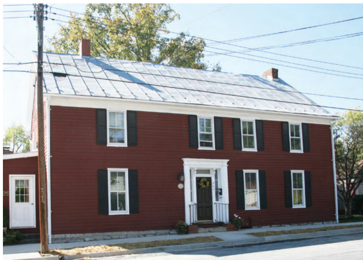
This vernacular residence has grown over time, likely with the later addition to the left in this image. Note the consistent larger windows on the first floor and smaller windows above. The windows are a late nineteenth century change as is the Italianate entrance feature.
