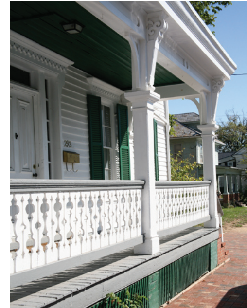
Scroll-sawn balusters complement the square posts and carved brackets of this porch set on brick piers.
