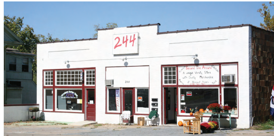
A variation on the illustration above, this one-story building is set back from the street and has three separate storefronts. Some of the multi-paned transoms that provided light to the interior have been covered, and the brick has been painted; but the building retains many original features.
