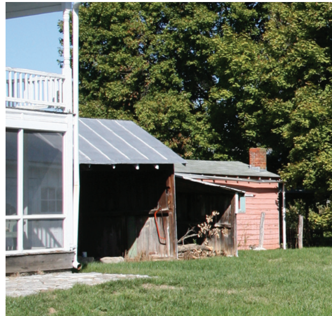
These outbuildings face into the rear yard and are likely to date to the period when town residents had to be self-sufficient, before the advent of automobiles and modern-day grocery stores.
