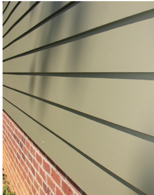
Cementitious siding can be applied to a new structure in the same manner as wood.
