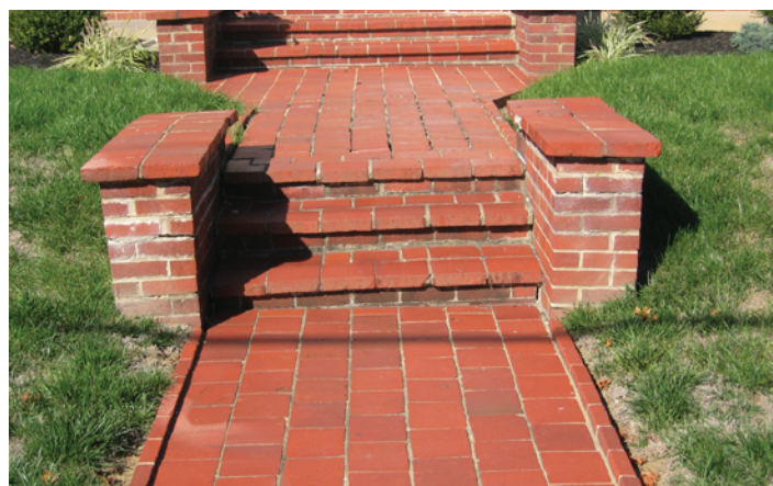
Brick is a common walkway material in the historic district. This walk is laid in an running bond pattern.
