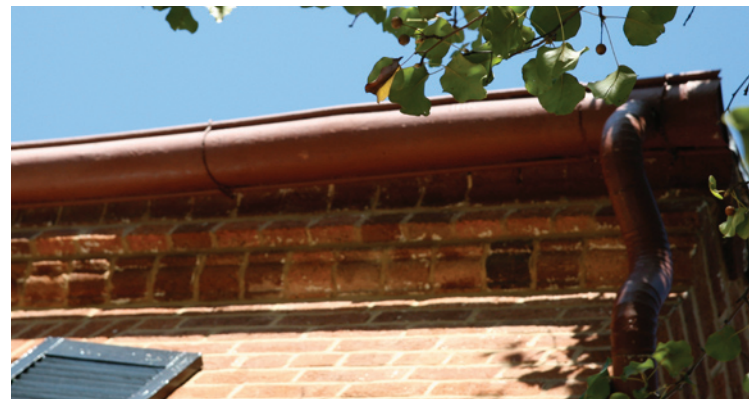
A brick mold cornice on King Street.
