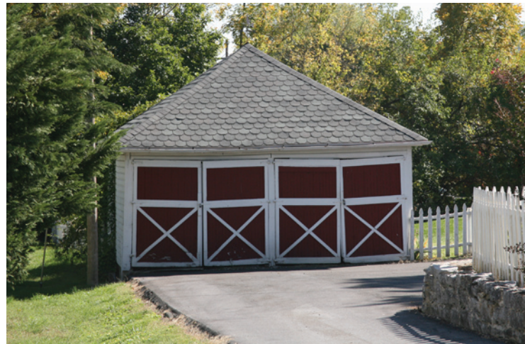
This garage has two pairs of doors with a more agricultural design.
