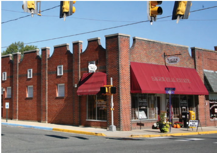
Among the examples of this style in the Old Strasburg Historic District is the Sager Real Estate Office, the former Virginia Restaurant, at 111 East King Street. The treatment of the shaped parapet divided into bays with simple pilasters is both decorative and unusual.
