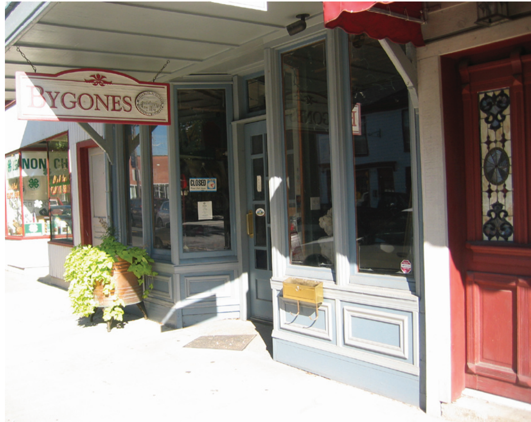
This King Street storefront has been well-maintained and many of its original features retained. The overhang of the second-story porch shades the plate-glass storefront windows which allow passersby to better see into the interior displays.
