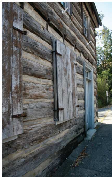
Rarely seen as an exterior surface, log construction may be present in a number of Strasburg's early dwellings
