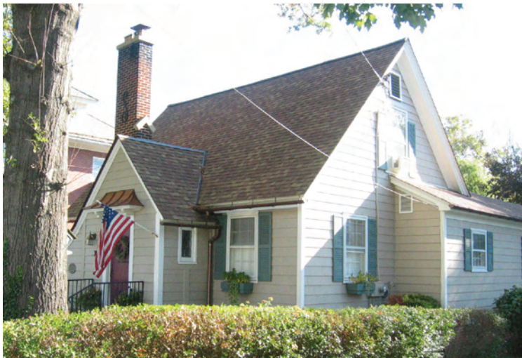
Note the steeply gabled roof and projecting cross-gabled entry bay of this siding-clad cottage.
