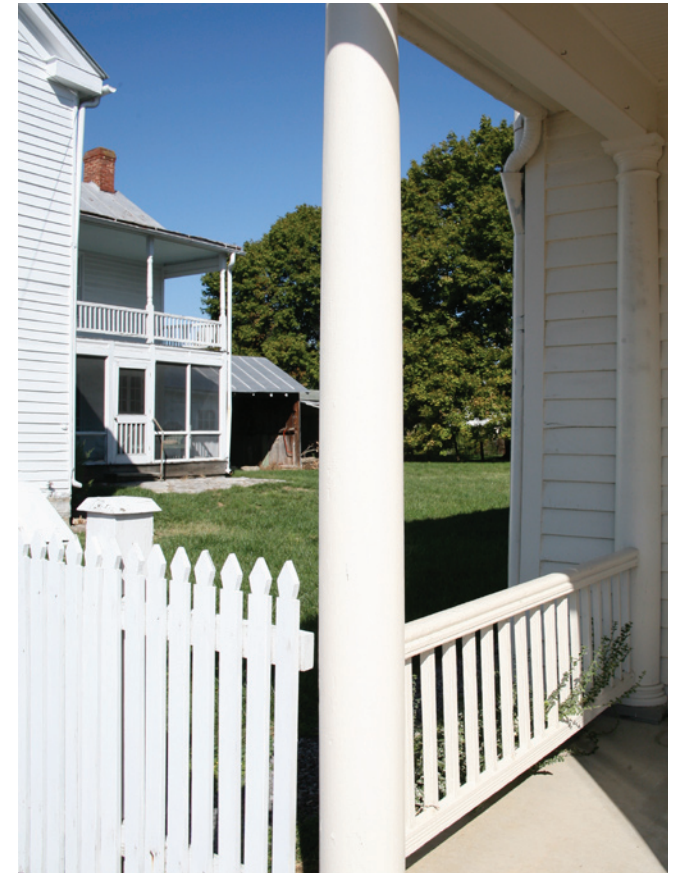
Two-story porches on rear ells, such as the one seen here, are a traditional design element to provide private outdoor living areas.
