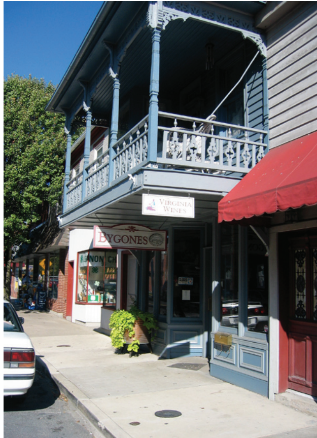
One of Strasburg's most unique features is the retention of historic second-floor gallery porches over a number of its historic storefronts on King Street.
