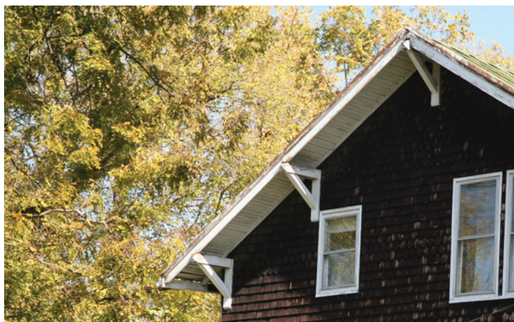
Deep overhangs show a Craftsman influence and are found on both Bungalow and American Foursquare residences in the district.
