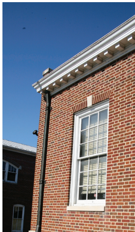
The classical modillion cornice is seen on both institutional and residential historic structures in the districts.
