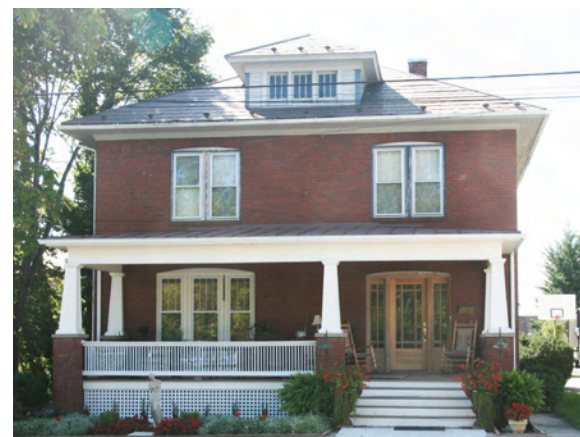
Paired or triple windows are often associated with the American Foursquare style as seen in this example. Also of note are the battered (tapered) porch columns that rest on brick piers. This features is often associated with the Arts and Crafts movement and seen frequently on bungalow style residences.
