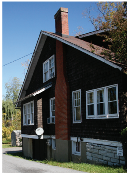
Late-nineteenth residences often incorporated centrally located chimneys with details such as the belt courses and corbeling seen here.
