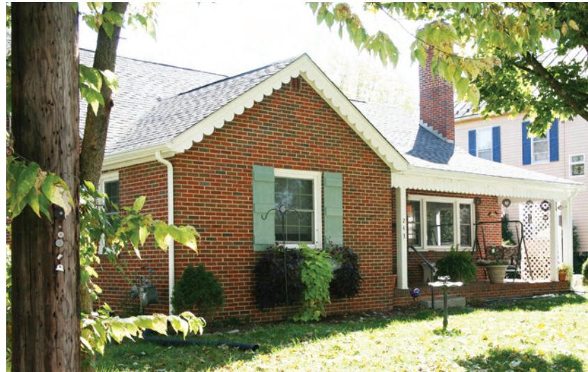
This one-story, Ranch-style house has a projecting front gable. Note the scalloped cornice on both the projecting gable and porch and the picture window under the porch roof.
