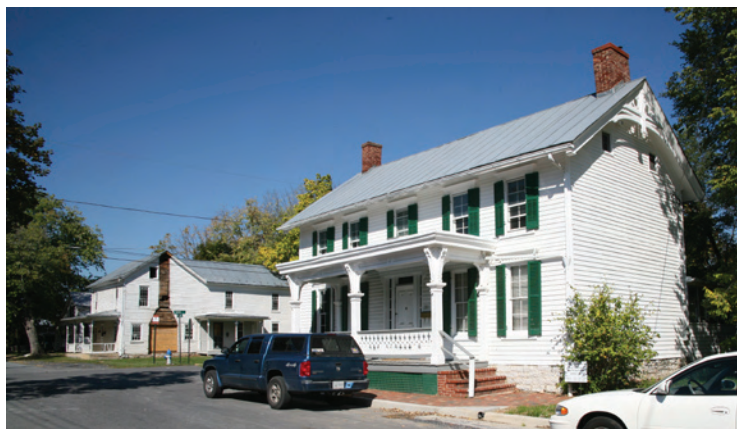
This symmetrically massed early-nineteenth-century frame residence on Queen Street was updated in the Italianate style. Note the window caps, scroll-sawn bargeboard in the gable end, and three-bay porch with bracketed columns and scroll-sawn balusters.
