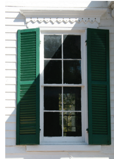
As technology improved, the pane size and window opening increased, leading to fewer panes of glass. The detailed decorative carving on the trim over the window is likely a later addition.
