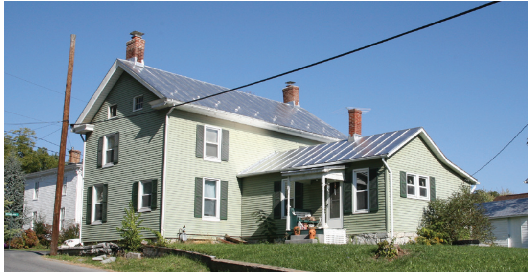
The one-story rear ell shares a similar roof form with the main portion of the house, however, the ridgeline is located well below the eave of the larger structure.
