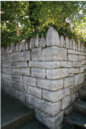
The uppermost course of stones has a jagged appearance, a style associated with a number of Strasburg sites.
