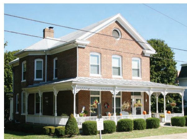
Note the intricately detailed porch cornice and round gable end window as well as the two-story side bay on this local example of a front-gable vernacular Victorian.
