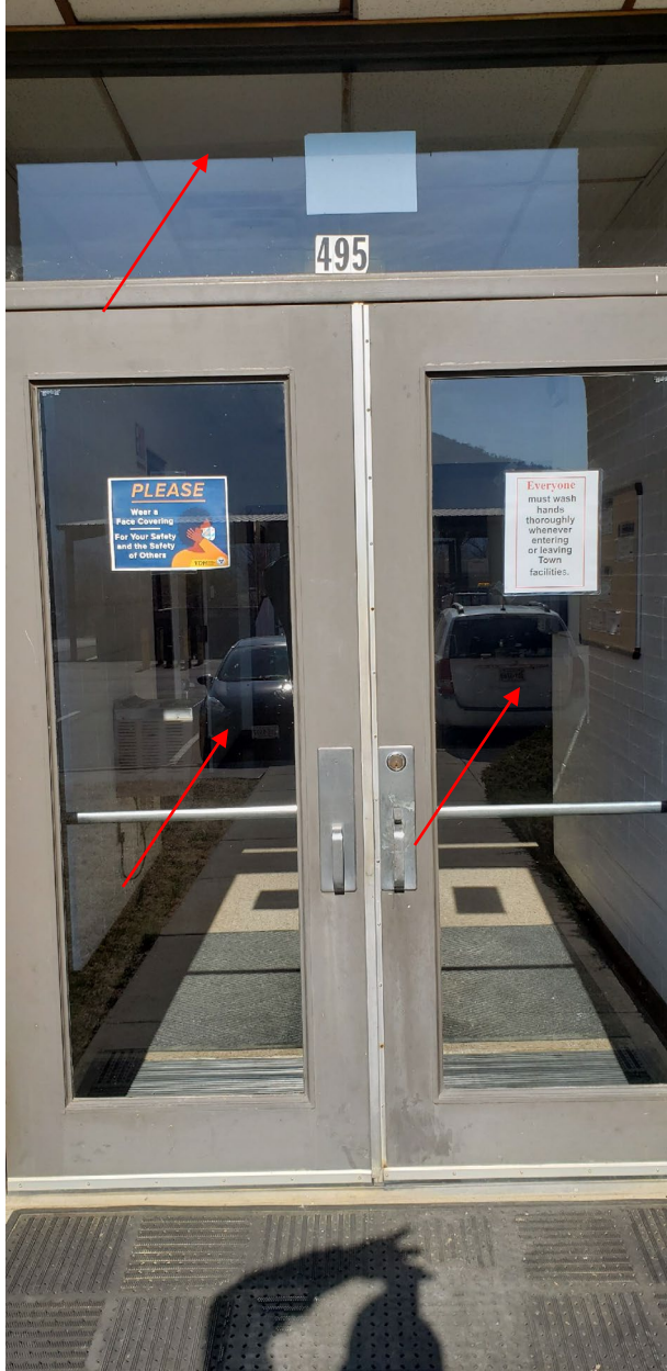
Figure 4 These are all single pane windows
