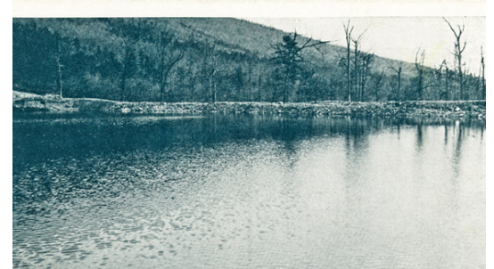
MUNICIPAL RESERVOIR, STRASBURG, VA. Signal Knob, two miles from Strasburg and the northern base of Massanutten range, is the end of two mountains. Diverging here, the two ridges form the shallow Little Fort Valley. Within this valley during 1922-23, the town of Strasburg constructed 900,000-gallon reservoir, a portion of which is shown above, and dug a 1,700-foot tunnel through Massanutten Mountain, through which the water flows to a 1,000,000-gallon supply reservoir on the town side mountain. The water is freestone, and the system, operating by gravity, is one of the finest in the Sta-
